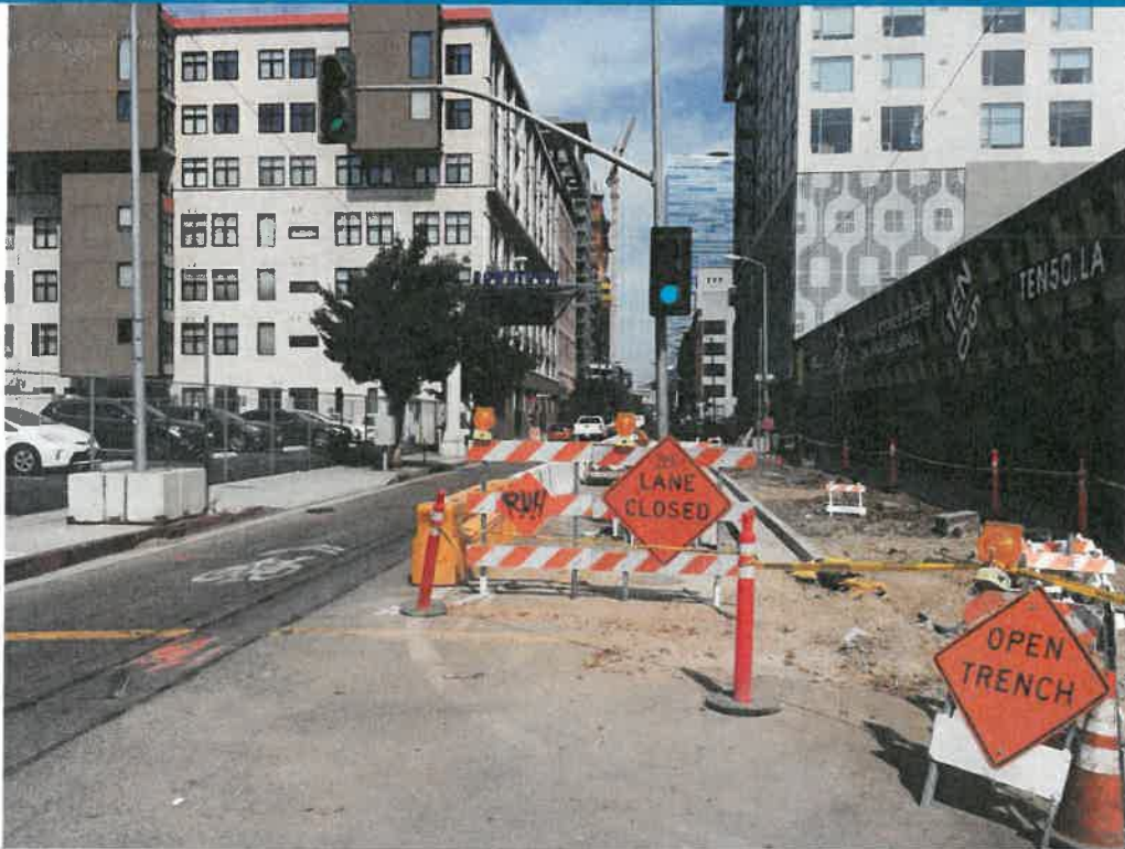
WESTERLY ORIENTATION ON 11 TH STREET
